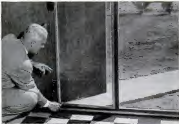
Cox operates a window opener that has been attached to panel in small unit built to serve as guest house or motel unit. Glass window panel at right is part of wall, does not open
